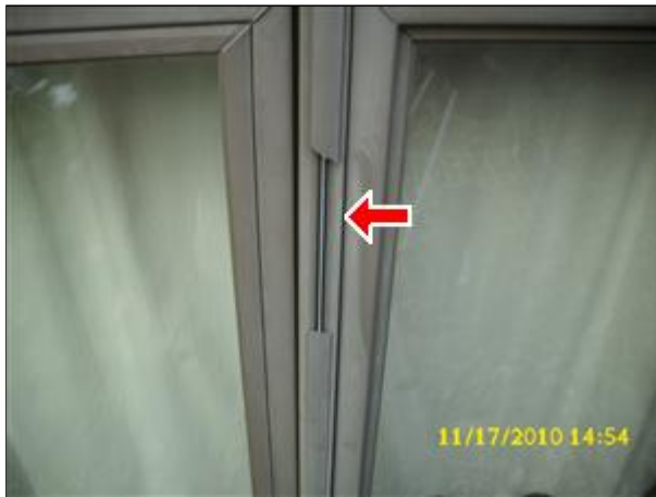
❌ (3) Missing glass stops observed on the patio door. Replacement is necessary to prevent water intrusion and to prevent the glass from falling out.
