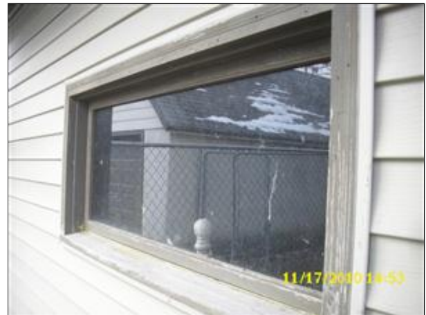
☒ (6) Deterioration of the paint/stain observed. Re-sealing is necessary to prevent further deterioration.
