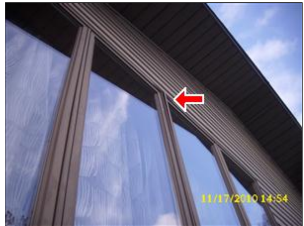
❌ (3) Missing glass stops observed on the patio door. Replacement is necessary to prevent water intrusion and to prevent the glass from falling out.
