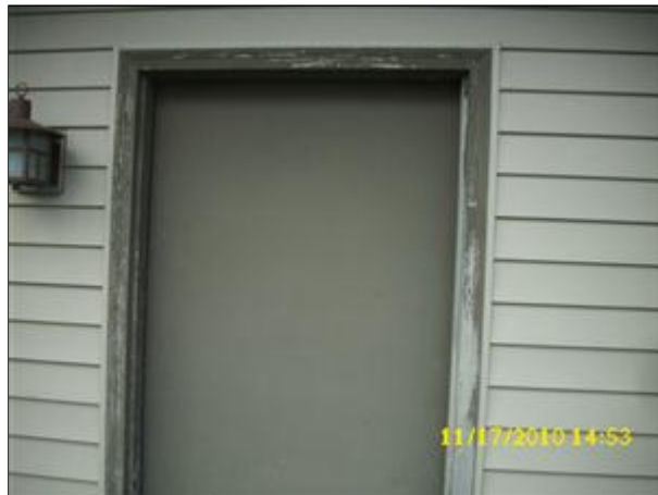
☒ (7) Missing mounting block observed for light fixture. Suggest correction.
