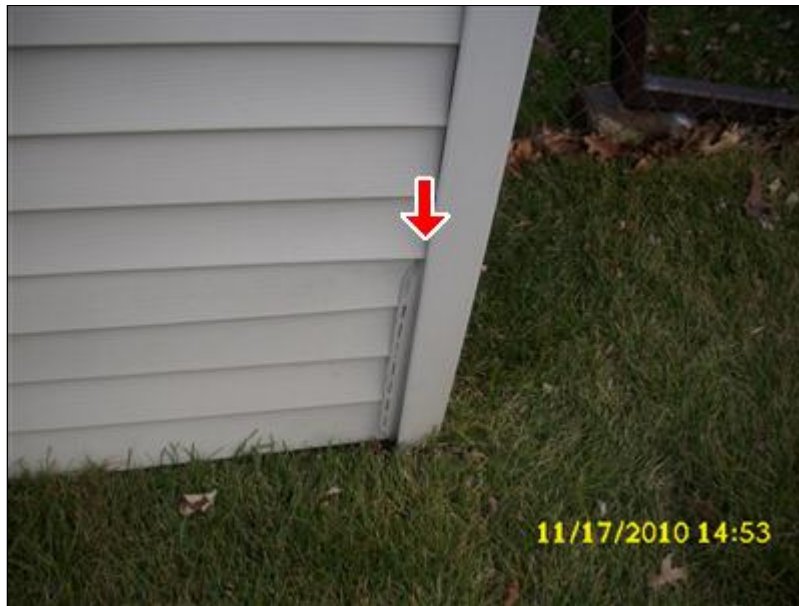
☒ (6) Deterioration of the paint/stain observed. Re-sealing is necessary to prevent further deterioration.
